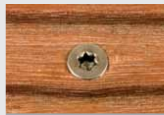
Pilot-drilling + Terrassotec screw
