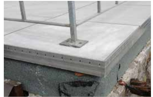
Example of application aluminium eaves
