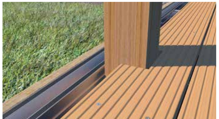
13 Saw notches for posts.
